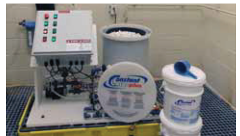
Little Egg Harbor Municipal Utility Authority serves 9,300 water customers. Drinking water comes from eight (8) main wells located at five (5) well sites. A Constant Chlor™ cal hypo system provides chlorination at one of these site.
